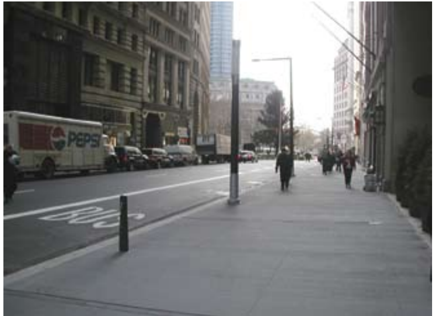
Typical tinted concrete sidewalk with simulated saw-cut joint scoring: Broadway at Exchange Place, Manhattan
