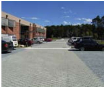
Permeable paving treatment used in a parking lot: Sutherland Shire, Sydney, Australia (Credit: Water Sensitive Urban Design)
