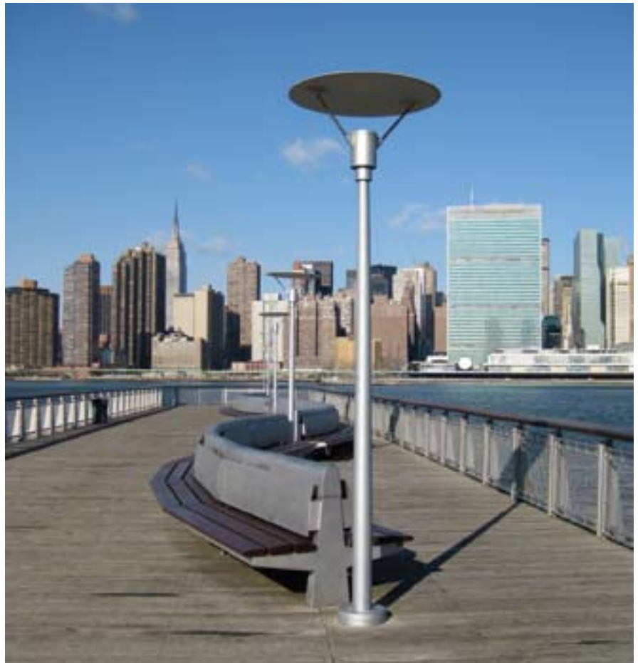
Round Top Head luminaire and pole: Gantry Park Plaza, Queens
