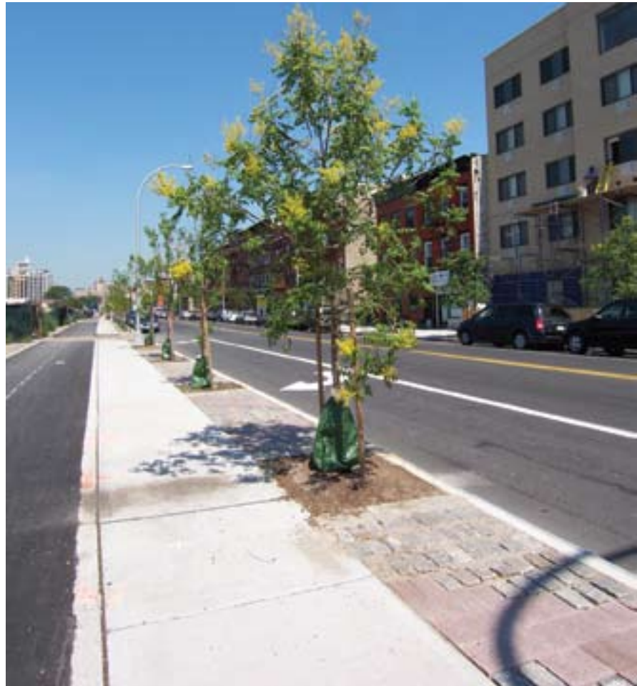
Connected tree pits with permeable paver-covered trench: Columbia Street, Brooklyn
