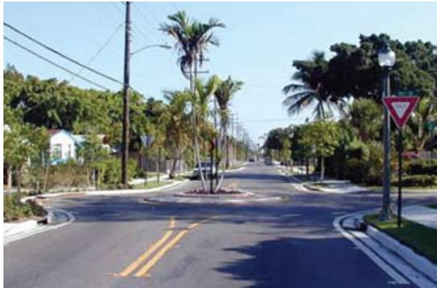
Neighborhood traffic circle with tree: West Palm Beach, Florida (Credit: Ian Lockwood and Timothy Stillings)
