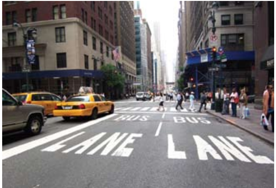
Curb-aligned double bus lane: Madison Avenue, Manhattan
