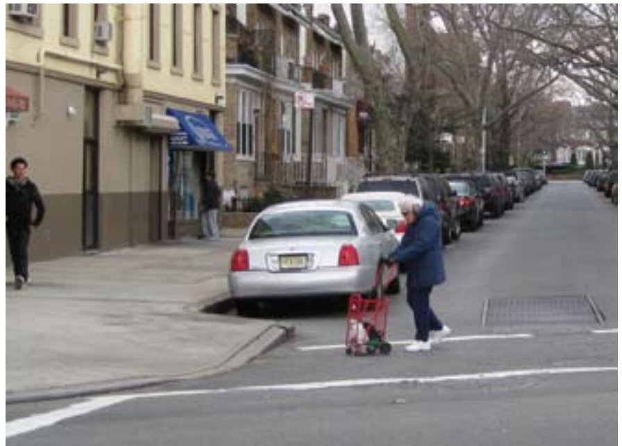
Curb extension: Fifth Avenue, Brooklyn
