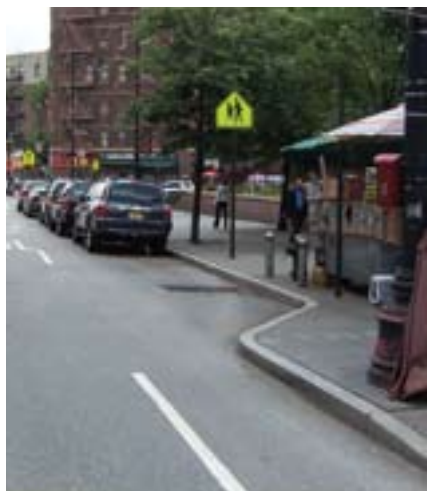
Curb Extension: Seventh Avenue, Manhattan
