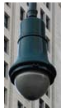
Historic Teardrop luminaire and Type F pole: East 8th Street, Manhattan
