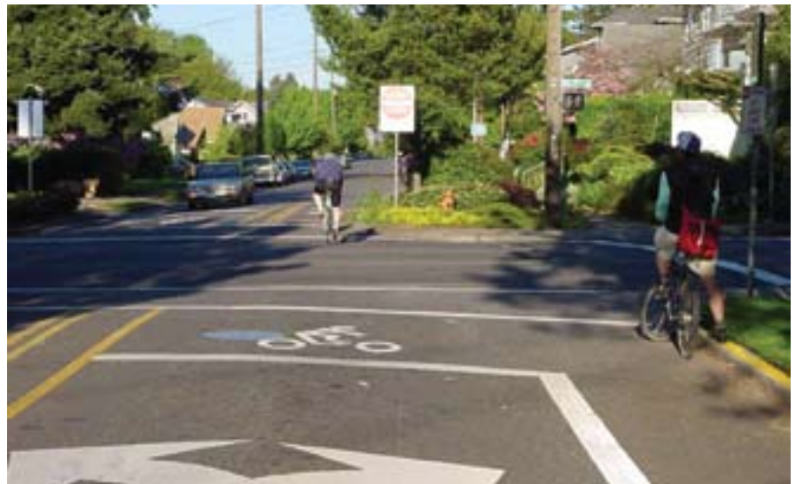
Half closure with landscaping and bike access: Portland, Oregon (Credit: Ryan Snyder)
