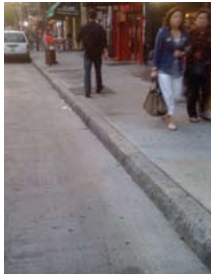
Split-finish granite curb shown with concrete sidewalk: Houston Street at LaGuardia Place, Manhattan
