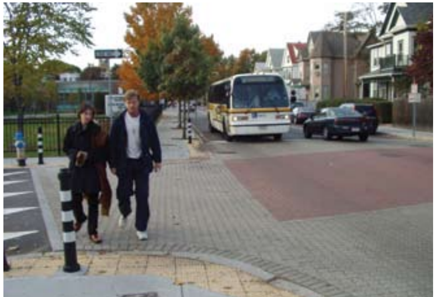
Raised Intersection: Cambridge, Massachusetts
