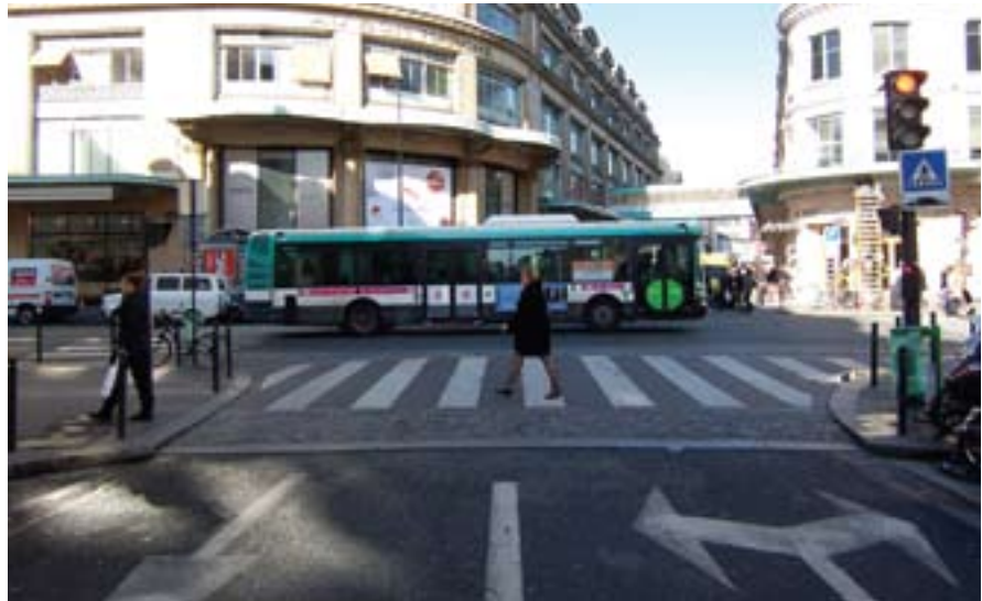
Raised crossing at a Gateway to side street: Paris, France (Note: for illustrative purposes only)
