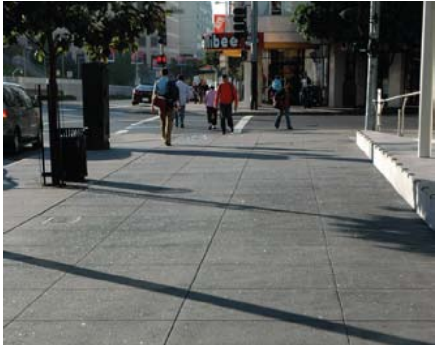
Tinted concrete sidewalk with silicon carbide treatment, shown with non-standard flag size: San Francisco, CA (Credit: Flickr user "Caribb")
