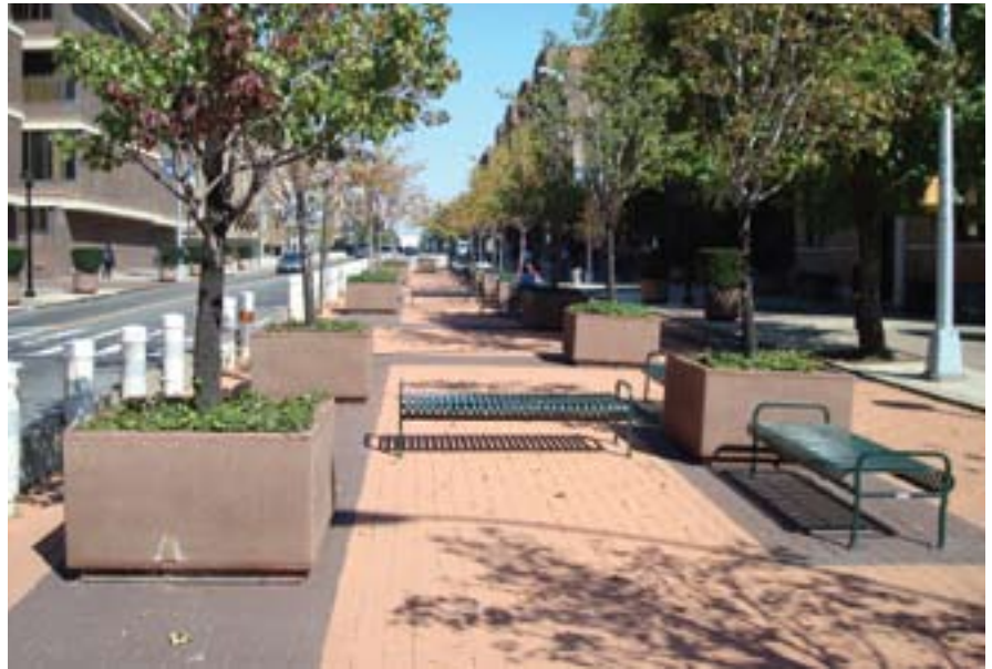
Imprinted asphalt pedestrian plaza in the roadway: 185th Street at Amsterdam Avenue, Manhattan
