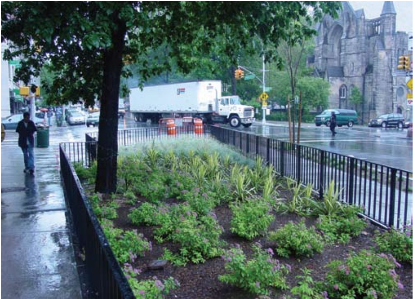
Greenstreet with stormwater-capturing design: Amsterdam Avenue, Manhattan (Credit: NYC DPR)
