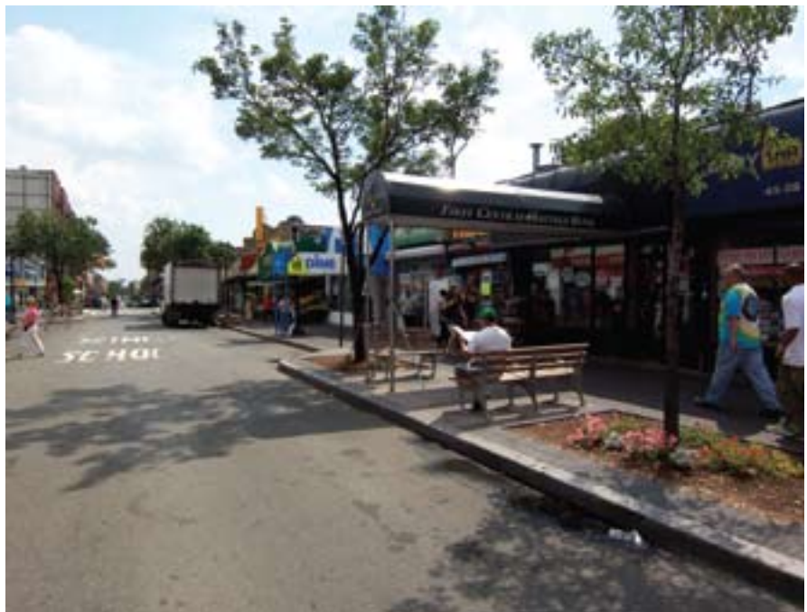
Curb extension with trees and bike parking: 46th Street, Queens
