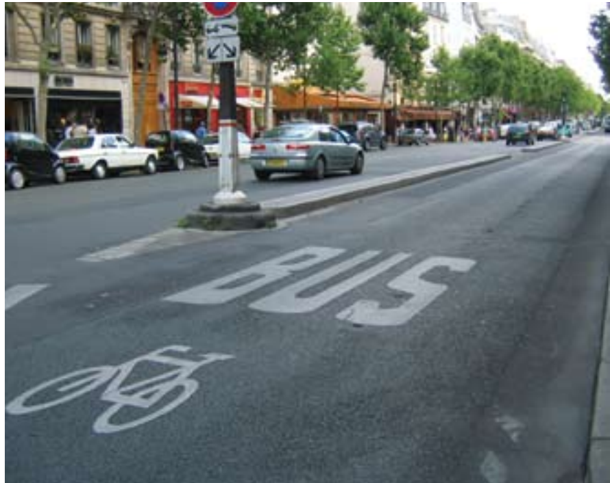
Curb-aligned busway: Paris, France (Note: For illustrative purposes only)
