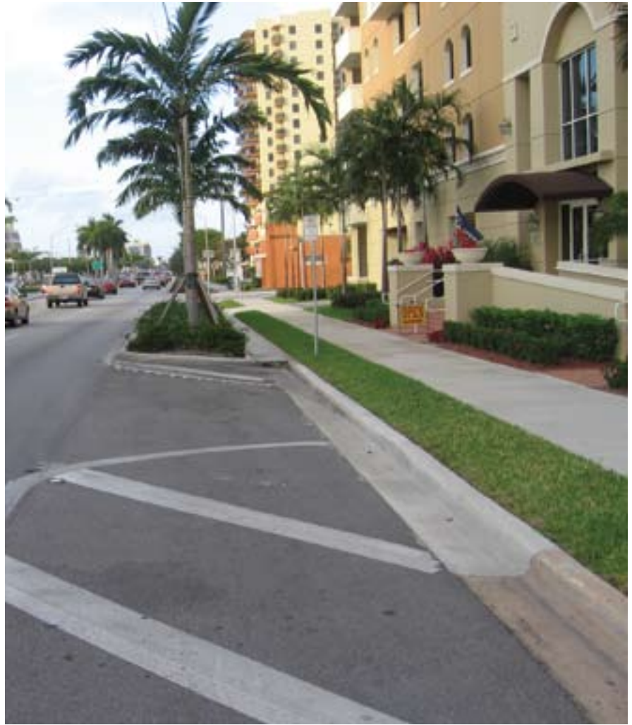
Precast concrete curb and gutter sections laid end-to-end. Photo shows optional sidewalk extension in background: Miami Beach, FL
