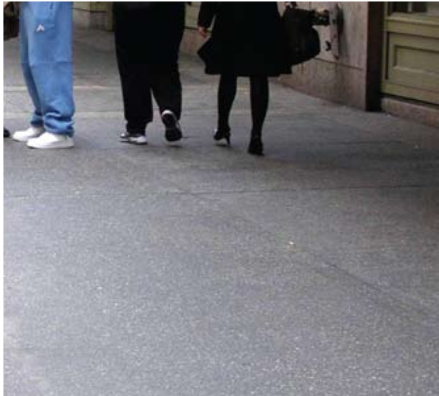
Tinted concrete sidewalk with light-colored exposed aggregate (note: this example does not include the required "simulated saw-cut joint" scoring pattern): 42nd Street at Grand Central Terminal, Manhattan
