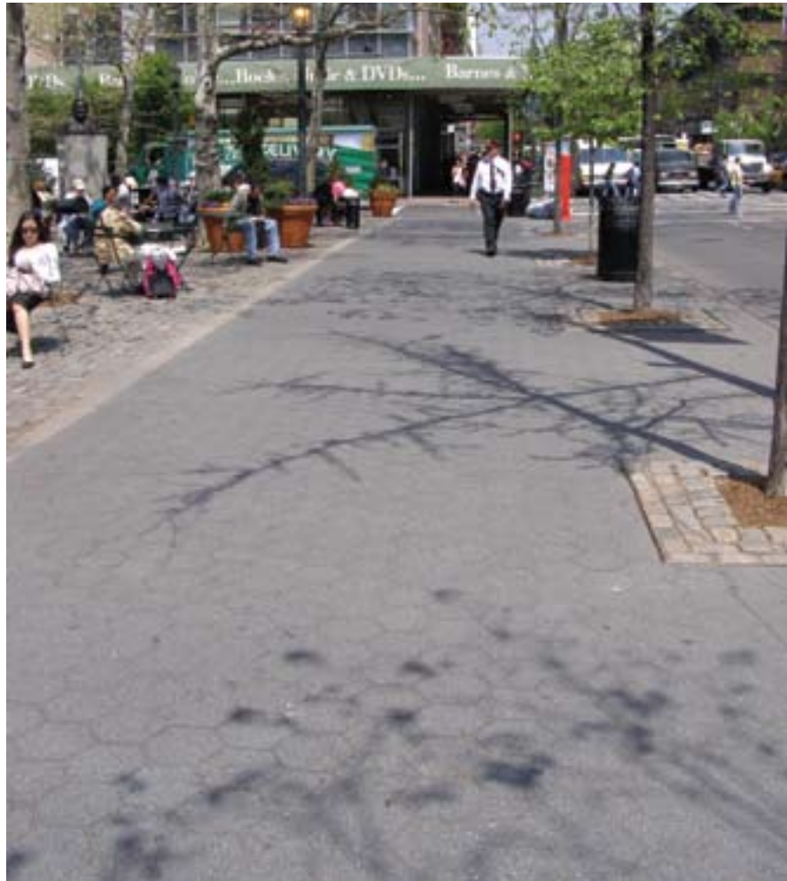
Hexagonal asphalt paver sidewalk: Columbus Avenue at West 66th Street, Manhattan
