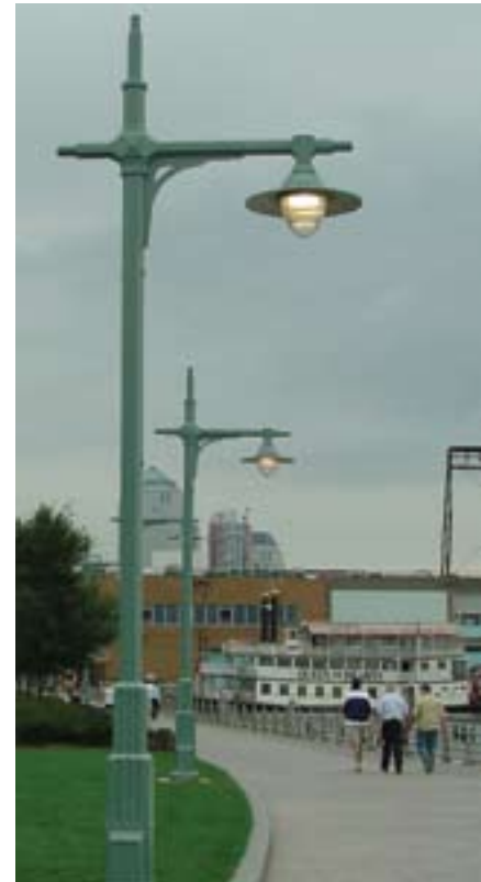
Historic Shielded Teardrop luminaire and TBTA pole: Hudson River Parkway, Manhattan
