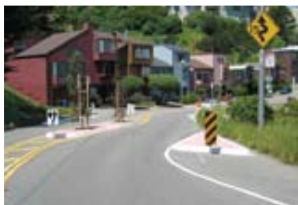
Chicane at entry to residential neighborhood: San Francisco, California (Credit: SF MTA)
