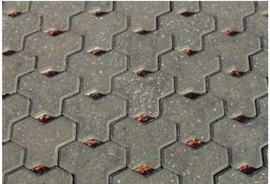
Voids between pavers allow rainwater to trickle through: Bicentennial Park, Sydney, Australia (Credit: Water Sensitive Urban Design)
