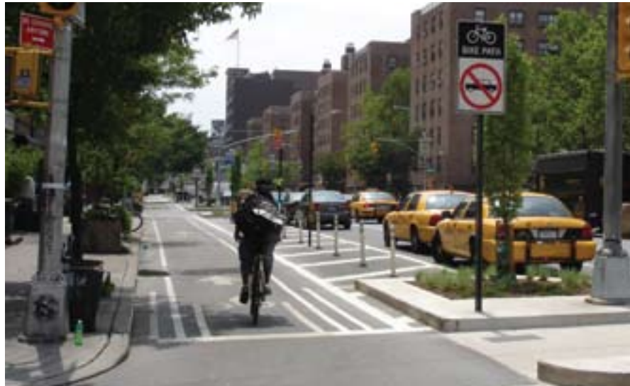
Wide, one-way, median-separated bike path on a busy avenue: 9th Avenue, Manhattan
