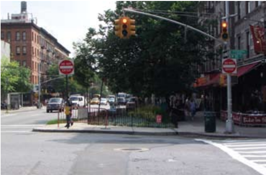
A curb extension “blockbuster” with Greenstreet: Amsterdam Avenue, Manhattan
