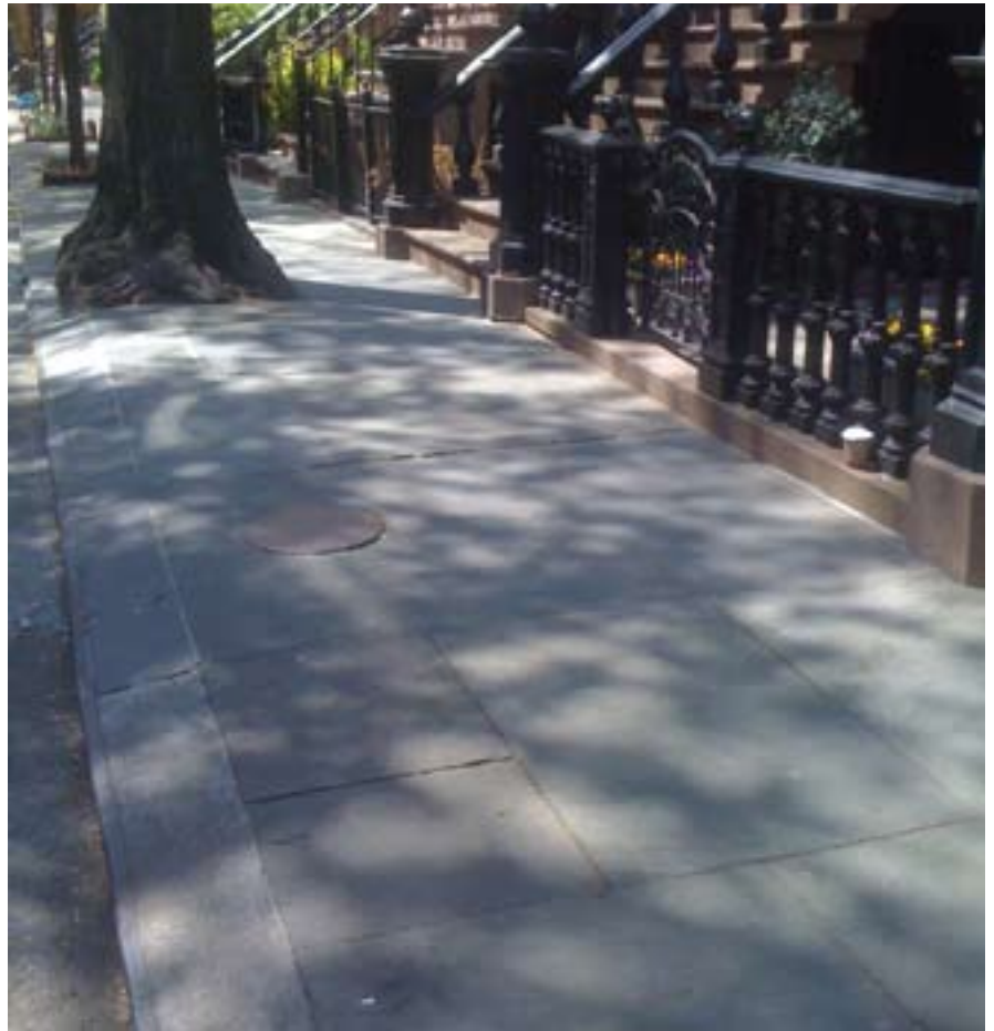
Bluestone flag sidewalk: Perry Street at Bleecker Street, Manhattan
