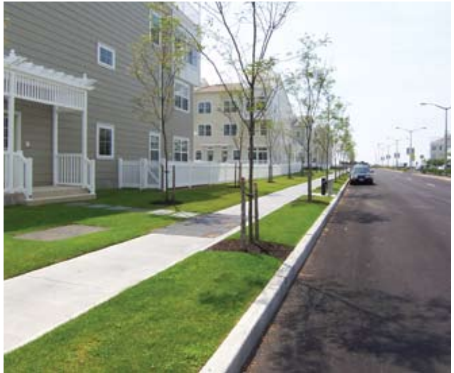
Typical concrete curb: Beach 73rd Street, Queens
