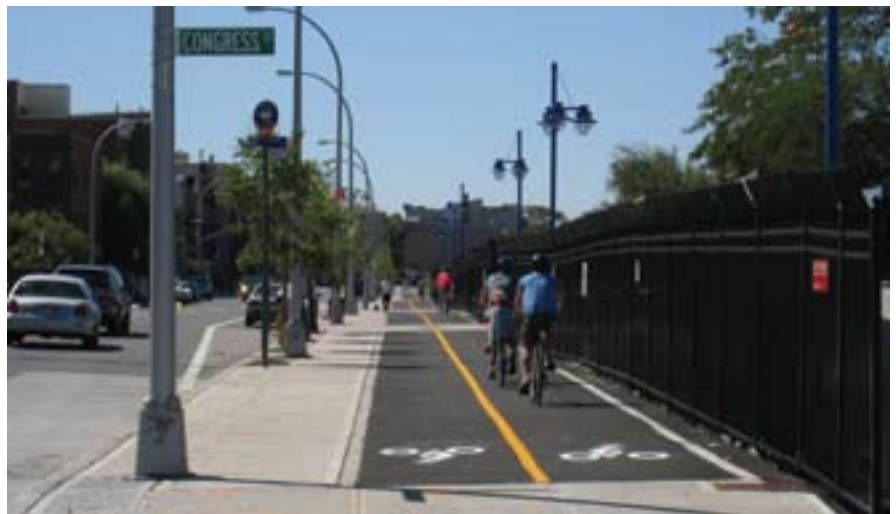
Two-way bike path located outside the sidewalk: Columbia Street, Brooklyn
