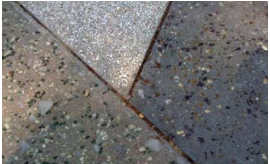
Poured, cast-in-place concrete with exposed glass aggregate: Brooklyn Plaza, Brooklyn
