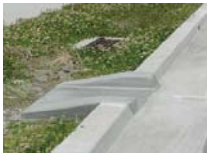
Street swale: Portland, Oregon (Credit: Portland Bureau of Development Services)
