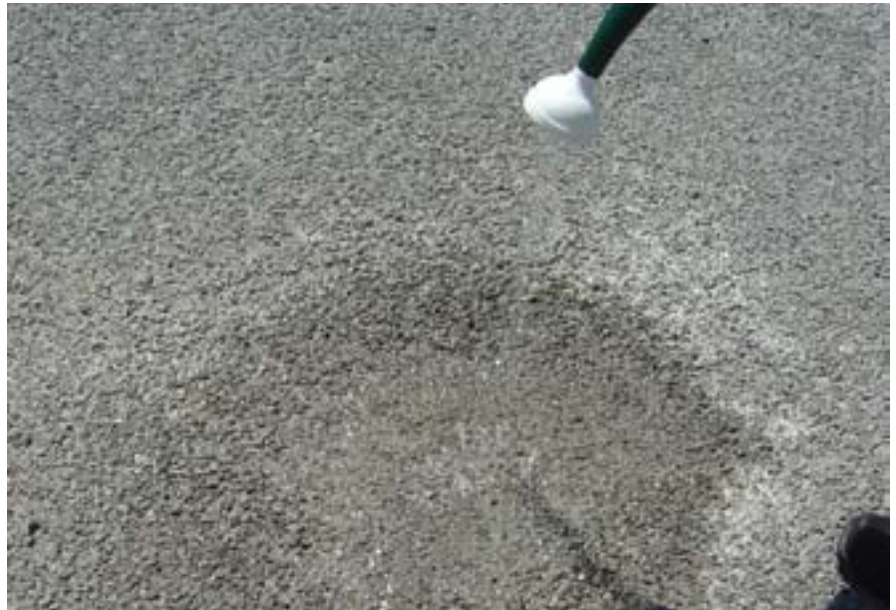
Porous concrete lets water permeate down to the subsurface soil
