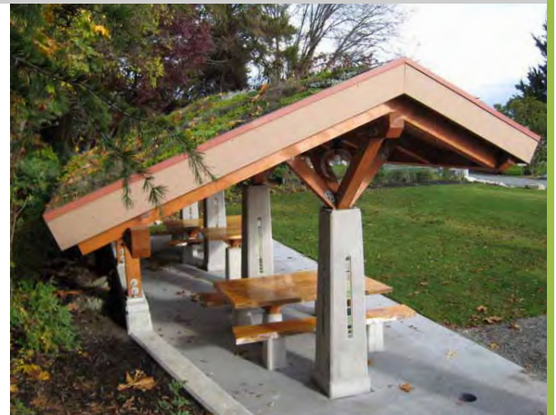
Green roof on picnic shelter
