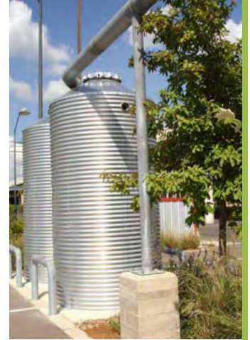
Collecting irrigation rainwater in old brewing tanks
