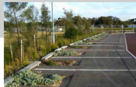
Treating stormwater with parking lot vegetation
