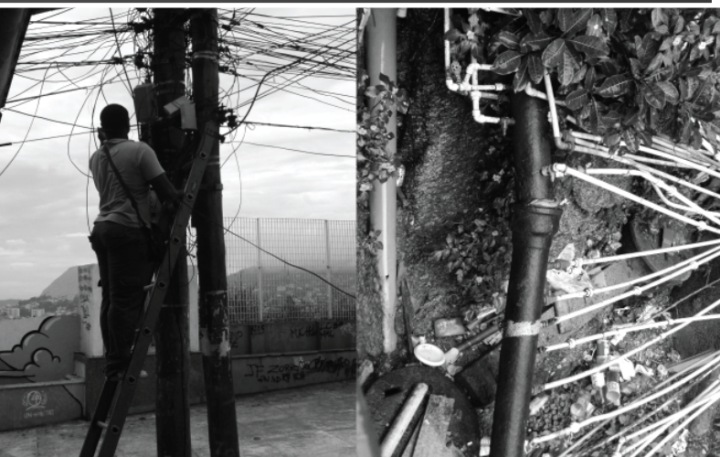
Image 5 - Informal plug in Morro de Providencia, Rio de Janeiro, Brazil. Although it is located in the center of the city, other borders prevent Morro de Providencia from being officially connected to the city's infrastructure. The inhabitants must informally plug in to access water and electricity.
