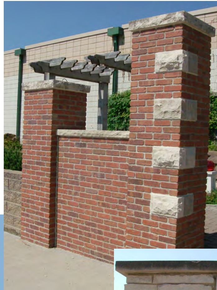
BRICK/STONE WALL AND COLUMN
