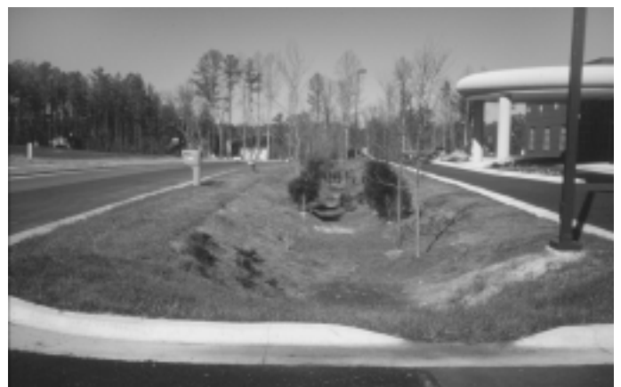
Figure 2. Bio-retention median in a Cary, N.C., parking lot. Bio-retention is a practical alternative for treating stormwater runoff from heavily impervious commercial areas.
