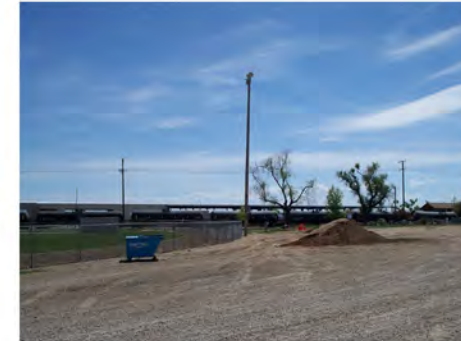
Existing railroad edge ^
