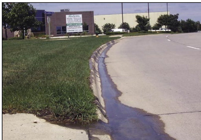
A hydrologically dysfunctional landscape. Water that can't percolate into the soil profile seeps out into the street two hours after a rain storm occurred.
