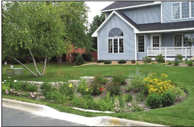
A rain garden with a backdrop retaining wall.
