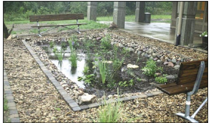
A rain garden in Okoboji has brick work edging and a mulch barrier.
