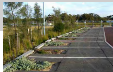
Treating stormwater with parking lot vegetation
